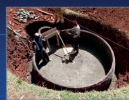
fermentation of the cow dung: biogas-installation for cooking on biogas in the Children's Home
